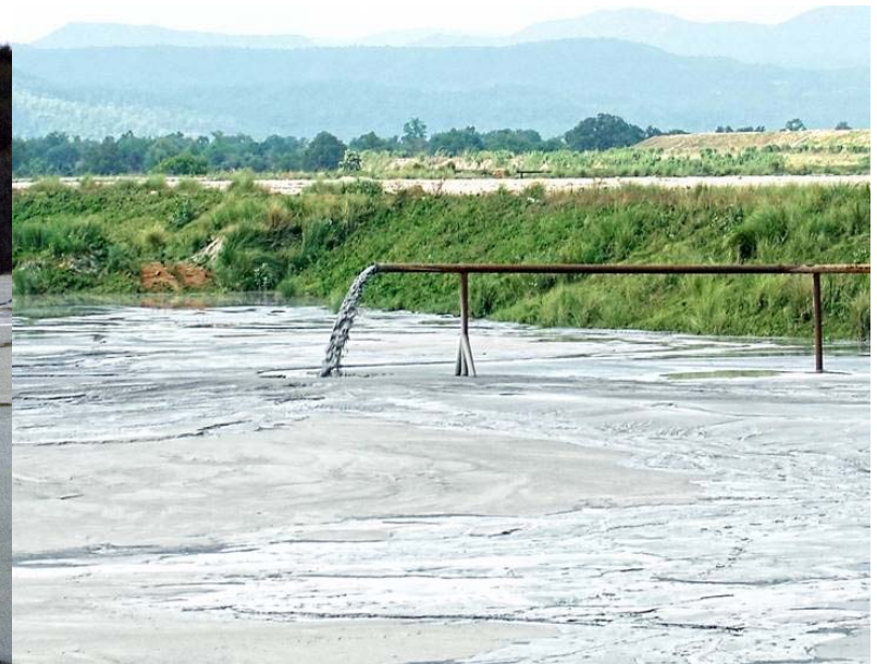
Example of ash being pumped into a basin
